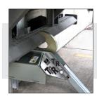
The TPR hook rotates up to engage the RIG and secure the trailer to the loading dock.
